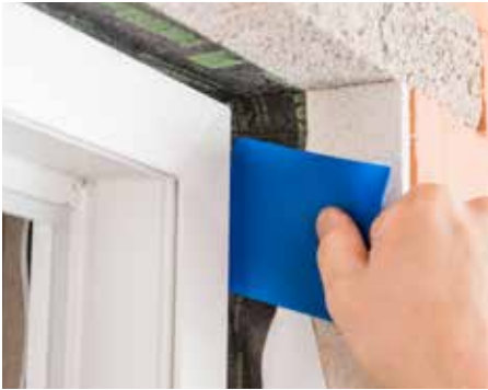
Tvirtai prispauskite PRESSFIX.
