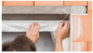
4. Apply masking tape to the window frame
