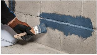
**5. Filling cracks up to 20 mm (0.8") in width** For cracks of 8 - 20 mm (0.3" - 0.8") in width, apply AEROSANA VISCONN FIBRE deep into the crack.
