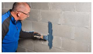
4. Painting over cracks up to 8 mm (0.3") in width
