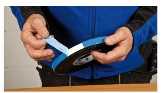
**2. Remove the protective film** Cut the outer protective film with a utility knife and remove this film.
