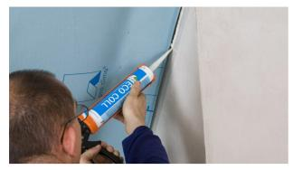
9a. Sealing to plastered chimney (insulated or double-shelled)
