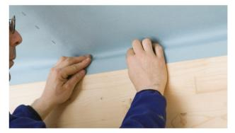
8b. Sealing to roughly sawn timber
