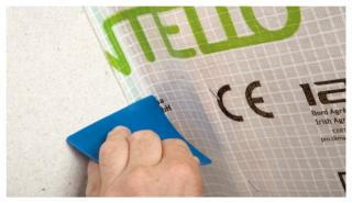
8b. Sticking the membrane / Rubbing the joint firmly
