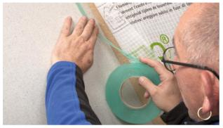
**8a. Alternative: Sealing to mineral subsurfaces** Position ORCON MULTIBOND on the subsurface, roll it out and gradually stick it to the subsurface. Gradually remove the release film.
