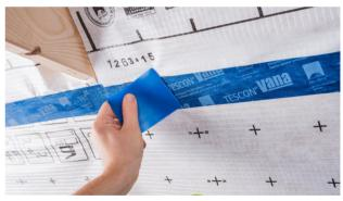
**5b. Rub the adhesive joint firmly** Rub tape firmly into place using the pro clima PRESSFIX. Ensure that there is sufficient resistance pressure.
