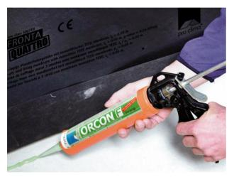
6a. Sticking to rough or mineral surfaces (e.g. floorboard)
