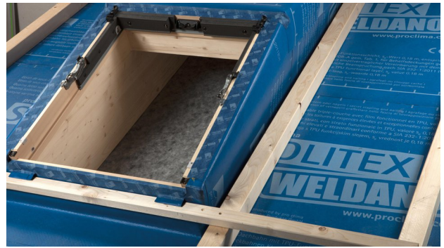
34. Install the counter battens and supporting battens, and screw the mounting brackets into place. You're finished!
