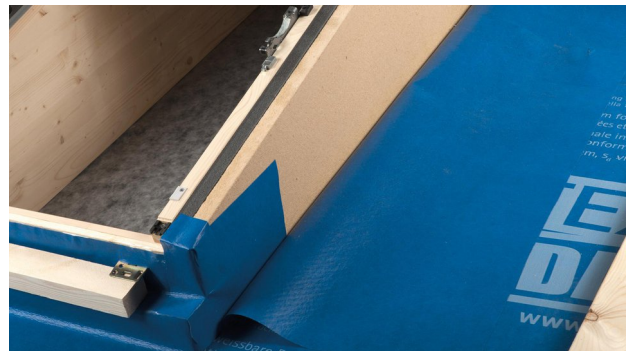
16. Finished bottom corner seal.
