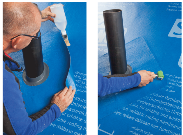
4. Weld the grommet to the membrane Weld the grommet around the edges using the WELDANO TURGA solvent welding agent or hot air. The effective joint width (area covered with solvent welding agent) must be at least 3 cm (1 3/16") wide and must extend as far as the edge of WELDANO ROFLEX PLUS. Use a roller to press the grommet in place.
