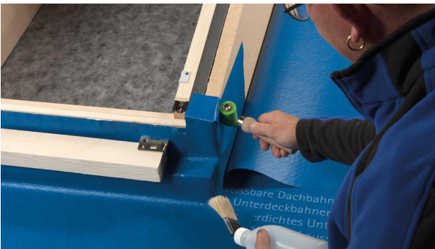
15. Fold the excess pieces and weld them to the lower membrane. Pay particular attention to ensuring the corners are sealed tight.
