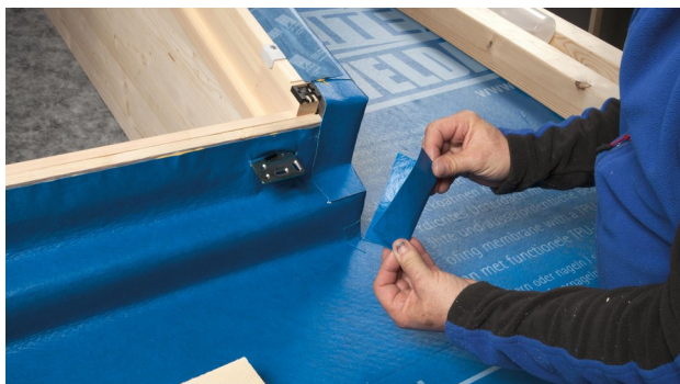
31. Remove the auxiliary supporting batten and cut out fitting pieces for sticking over the mounting brackets.
