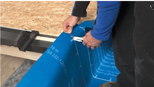
17. Guide the membrane from the main surface onto the side of the wedge-shaped frame. Alternatively, cut a new strip of SOLITEX WELDANO 3000, guide it up along the wedge-shaped frame and weld it at the bottom to the flat membrane.
