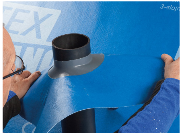
2. Create the bond Guide WELDANO ROFLEX PLUS over the pipe.
