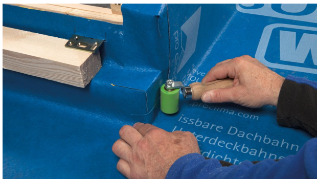
29. Weld the strip of SOLITEX WELDANO 3000.
