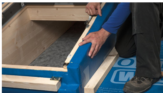
22. Stick SOLITEX WELDANO 3000 onto the edge of the frame. Put the membrane in place on the adhesive bed, leaving slack to allow for expansion. Do not press the adhesive completely flat so as to allow for relative motion between components.
