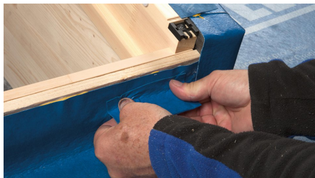
32. Enclose the mounting brackets by means of welded bonds.
