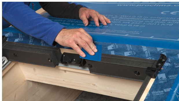
26. Use TESCON VANA for practical fastening of the installation.
