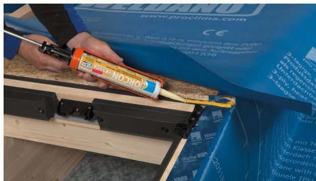
24. Stick the main sheet of SOLITEX WELDANO 3000 to the top of the window frame using ORCON CLASSIC.
