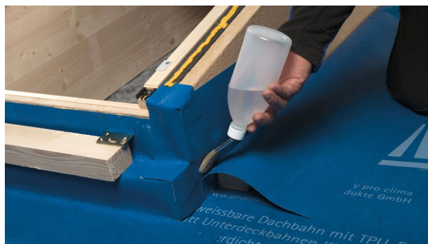
20. Weld the lower corner area.
