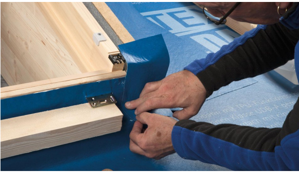
13. Ensure that the fitting piece fits well into the corners.
