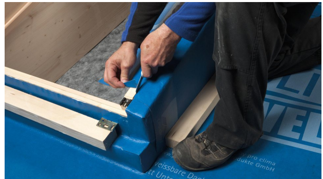
18. Cut to size parallel with the window frame. An auxiliary batten can be used to help affix the lower edge without folds or creases.
